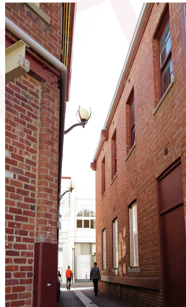
Heritage buildings, Wolf Lane, Central Perth
