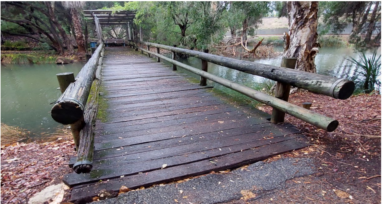
Figure 1: John Oldham Park – Timber Bridge
