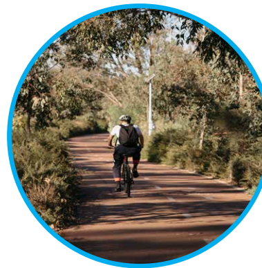
Limited sight lines
