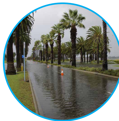
Recent flooding Riverside Drive 2020
