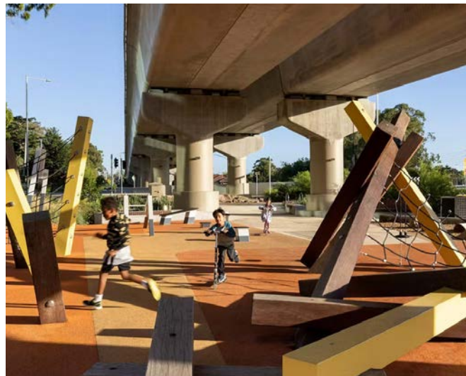
Toorak Road Level Crossing Removal Project , Melbourne, Aus
