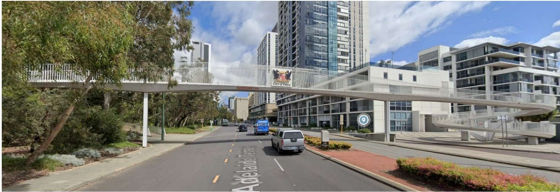
Figure 2: Adelaide Terrace Pedestrian Overpass Bridge
