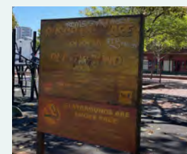
Bore water staining
