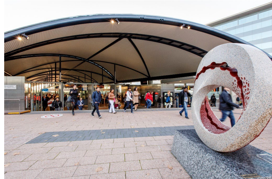
Figure 2-13 Elizabeth Quay railway station
