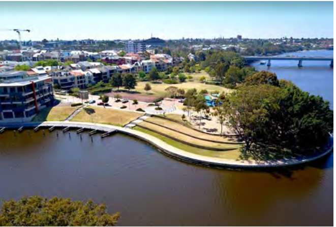
Grassed terracing providing premium outlooks over Swan River, back towards the cove & towards Optus Stadium
