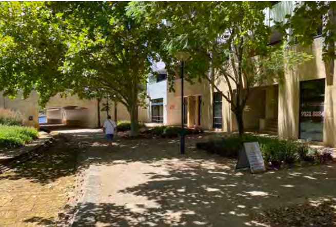
Uneven pedestrian thoroughfares due to existing trees lifting paving
