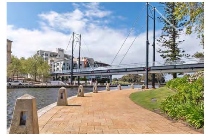
Consideration required to path width & safety along cove edge
