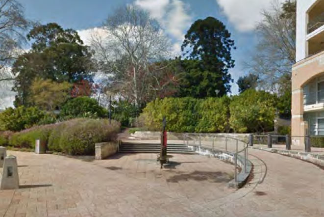
Stairs are located at the base of the bike path creating safety & clashing issues
