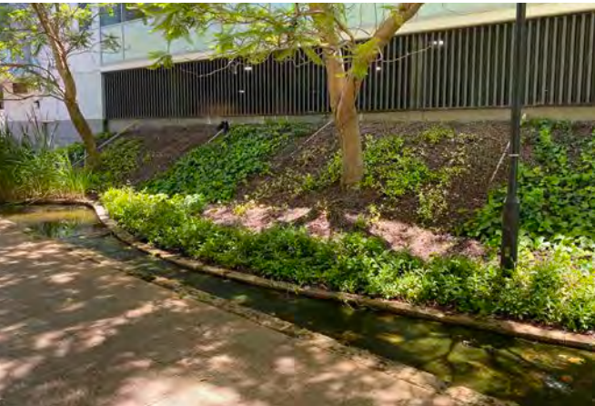
Algae build up to water feature. Lack of water movement in this area & shade from trees
