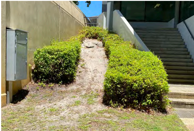
Degraded landscaping to batters. Replace with more suitable landscape response
