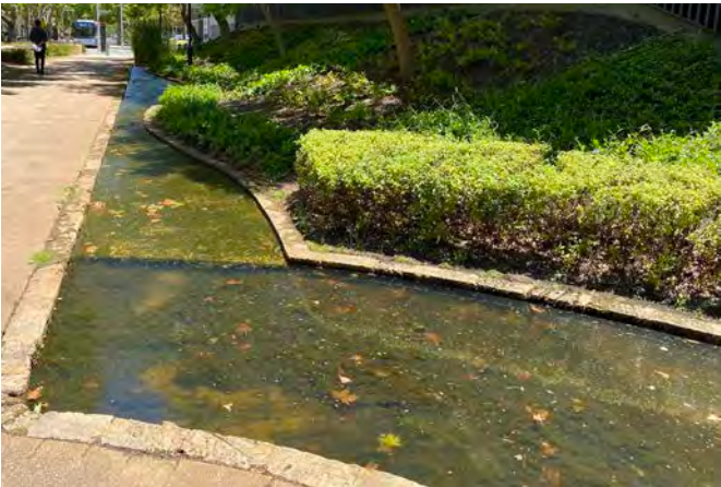
Algae build up to water feature. Lack of water movement in this area
