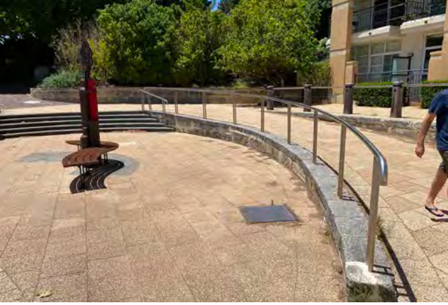
Ramps are disjointed & create pedestrian safety risks with bikes
